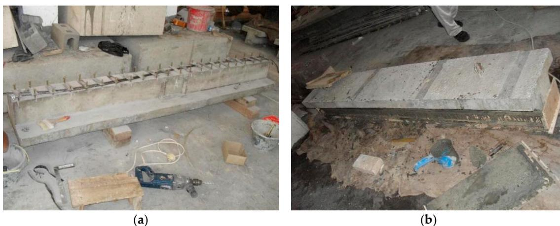
**Figure 2.** Strengthening system: (a) FC-SWRs fastened with steel plates and dynabolts; (b) mortar adhesive.
