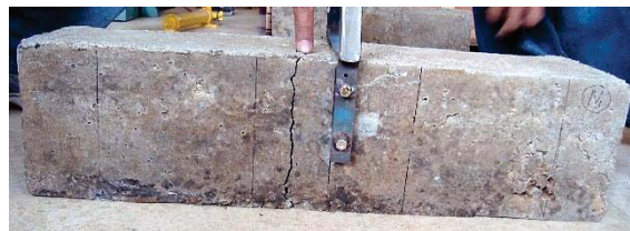
FIGURE 7. Failure mode on ALWA with fiber concrete occurred with the flexural failure mode in the beam's middle span.
