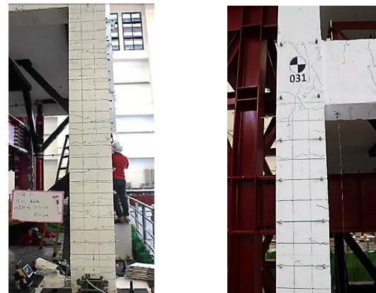
(d) The damage on the column and BCJ component from the experimental program
